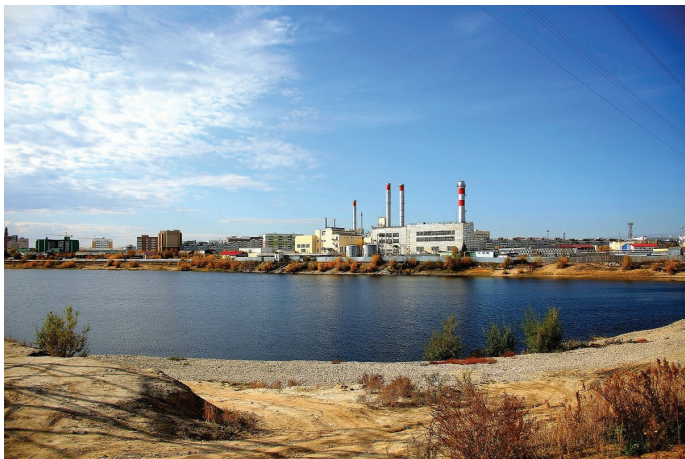
Рис. 1. Вид на пруд-охладитель Якутской ТЭЦ [6] Fig. 1. Cooling pond of the Yakutsk combined heat and power plant (CHP) [6]
